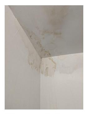
Photo 2 – Room #18 back office/kitchen area, possible visible mold growth was apparent on the wall and ceiling. AEG recommends removal of the wallboard during controlled renovation/demolition services. It is recommended that the roof above the ceiling be inspected by a roofing professional to address the root cause of the water incident.
