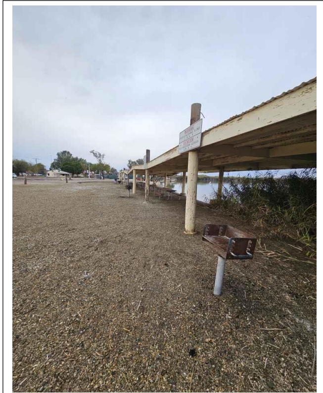
1. Area of shade structures to be replaced; sparse phragmites looking south
