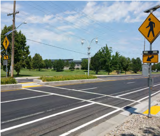
Rectangular Rapid Flashing Beacon (RRFB) with a Painted Crosswalk
