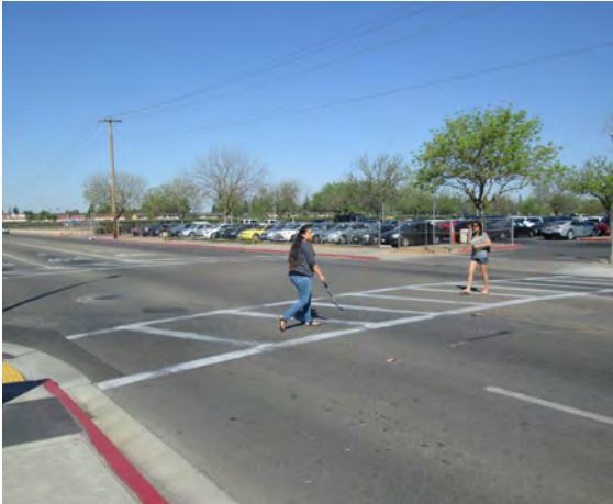
Continental Crosswalk with ADA Curb Ramps
