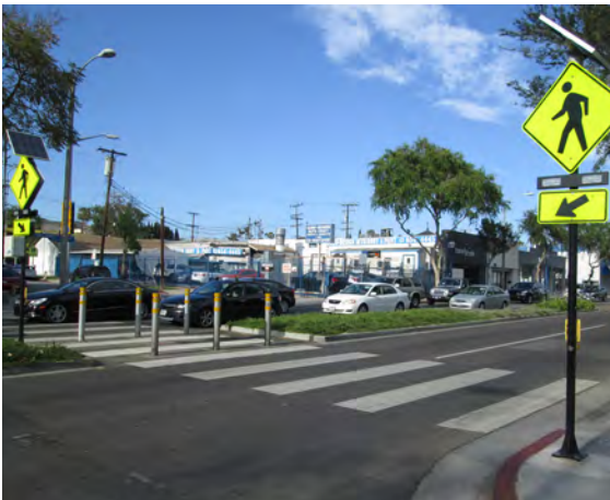
Rectangular Rapid Flashing Beacon (RRFB) with a Continental Crosswalk
