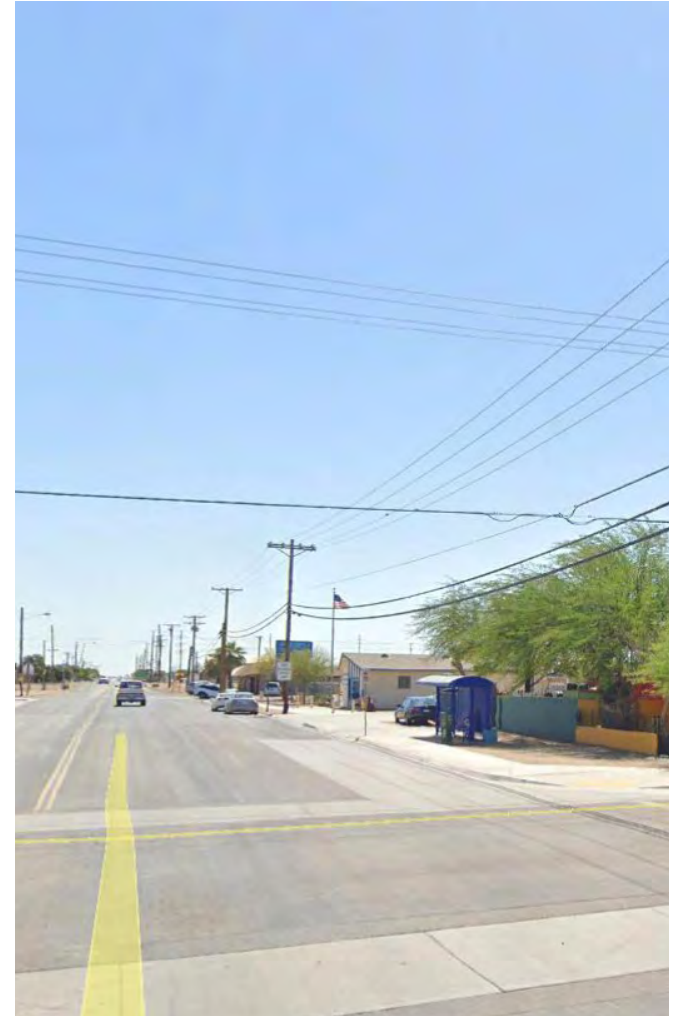
Intersection of Heber Rd & Parkyns Ave looking east Source: Google Earth
