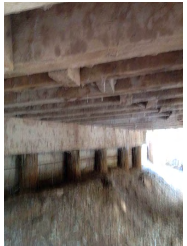
12. East side of the New River Bridge looking west.
