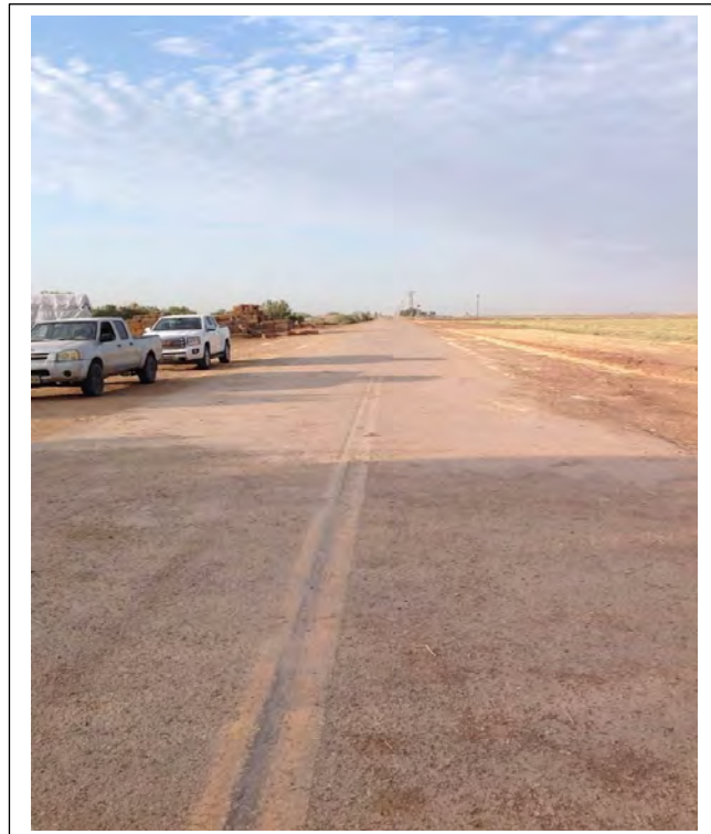
3. South end of the New River bridge looking south on Lack Rd.
