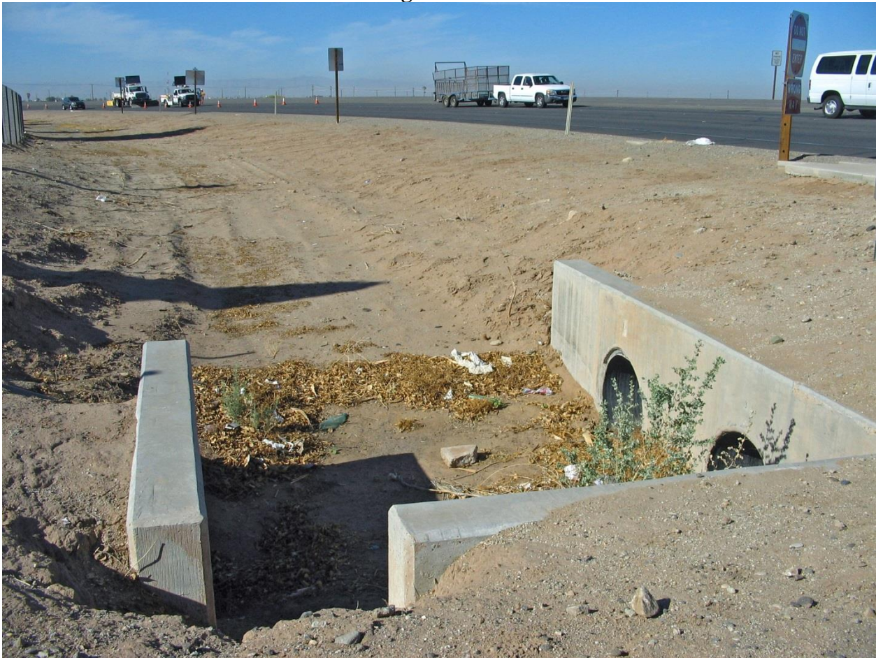
Existing drainage facility at the southwest corner of State Route 7 and Menvielle Rd, facing southwest
