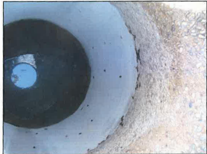
Typical concrete corrosion found within the cone of many of the CCSMD manholes. The concrete cone on the right should be smooth with no exposed aggregate, similar to the section below.
