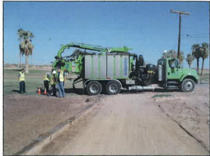
Vactor truck cleaning operations at newly located MH 7 within the golf course. Note the size of the equipment required to efficiently maintain the system.
