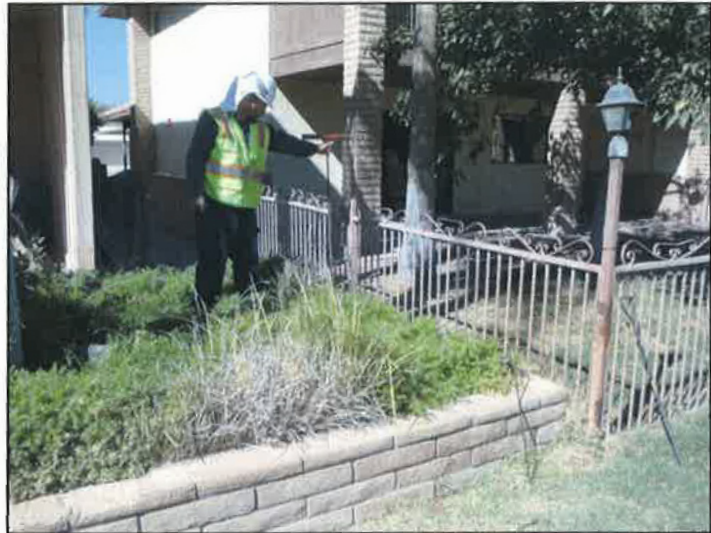
The worker is holding the probe at the center of MH 29, which is in a private backyard underneath the decorative wall on the left and the wrought iron fence on the right.
