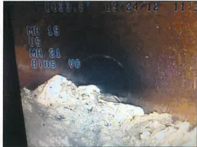
Image taken directly from CCTV camera shows an 8-inch pipeline between MH 19 and 21 that is 25%+ full of silt and debris.
