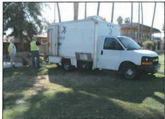
Video inspection operations at MH 26. Note the location of the manhole and sewer line at the rear of the van within private backyards; this is one of the more accessible locations.
