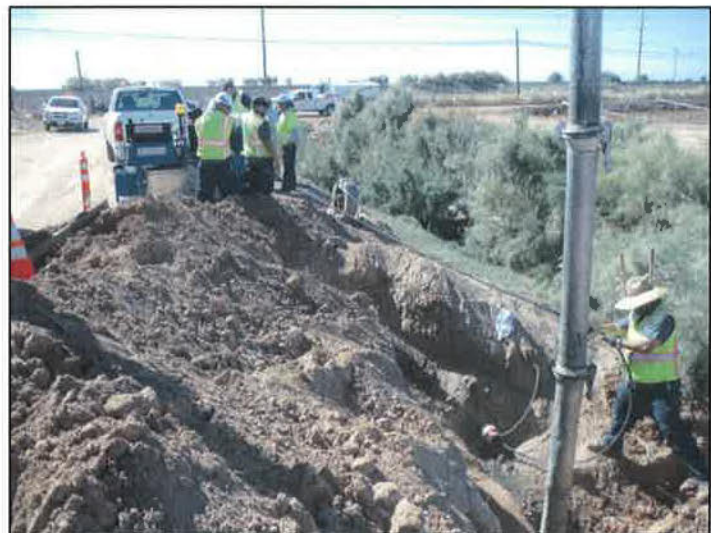
Second video inspection of the force main along Barbara Worth Drain, pump station is in the left background. The end of the pipeline can be seen in the trench, one line in the pipe is the video cable, the other is the jetter line used to pull the camera into the pipe.
