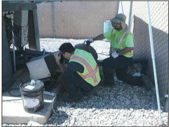
Initial video inspection of the force main with a push camera. Pump station is on the left and force main is on the right. Note the sharp 90-degree bend in the force main next to the fence.
