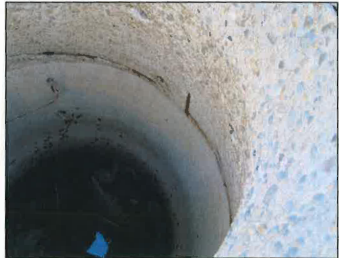
Manhole 5 showing corrosion.
