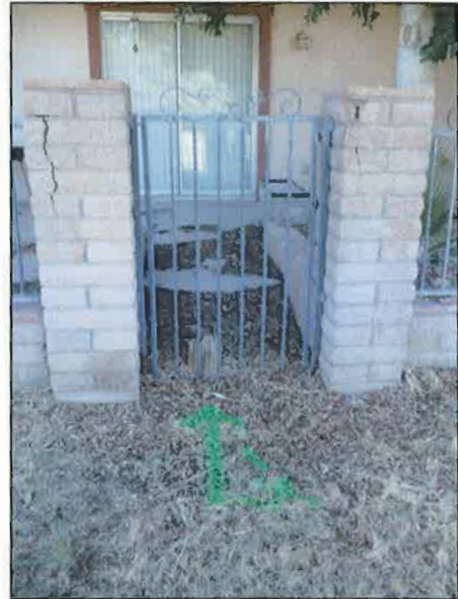
Location of MH 25 within a private patio, as located by the video camera with a tracking device.
