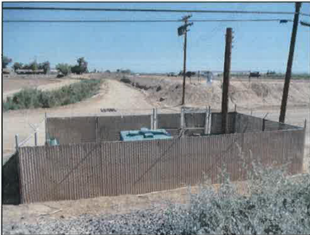
Wastewater pump station
